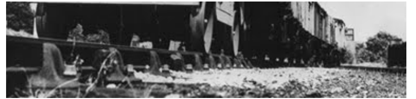
To illustrate the extra pulling power with the new diesel engine in 1962
