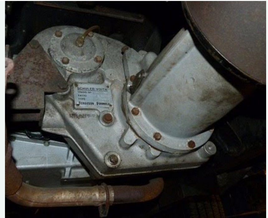
Larger picture of the number #488 Schuler FF transmission
